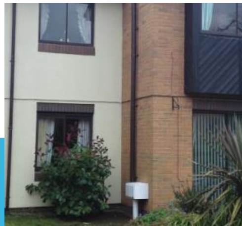
Install a radon sump system
