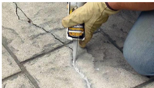
Sealing floors, walls & cracks
